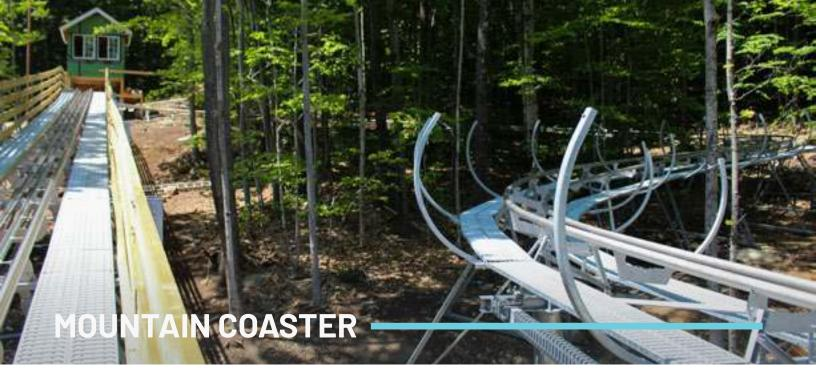
Mountain Coasters have quickly become a financial anchor for summer operations at ski areas of all sizes. The ride is equivalent to a one cart roller coaster that runs on a steel railed track. Riders load at the bottom of the ride and are pulled up the track to the top, where gravity takes over, propelling the cart down.
